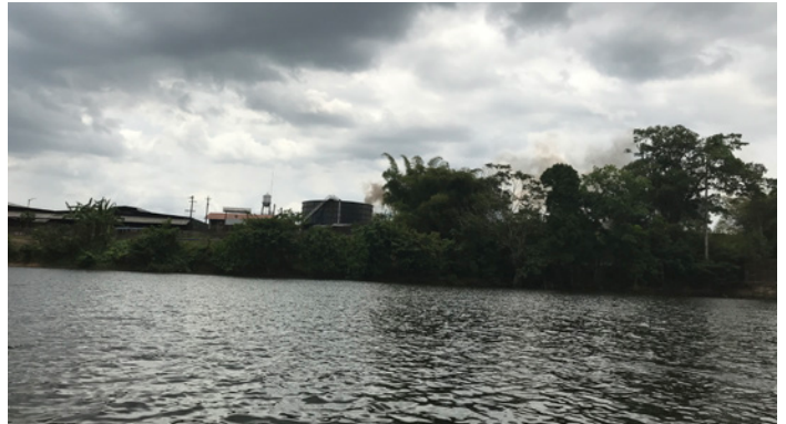
Firestone's existing wastewater facility
