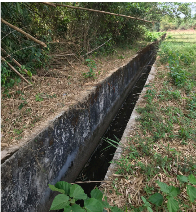
Wastewater channel running out from the Firestone factory
